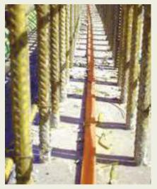
AMROCK Hydrophilic swell bars play a vital role in construction joints, swelling at the center of the joint post-construction when encountering water from leaks. This expansion effectively seals off any potential leakages, ensuring robust watertightness in the structure.
